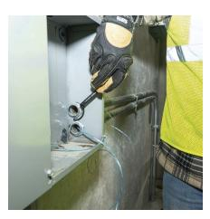
"Klein Tools' new Locknut Wrench Set is designed to make loosening and tightening locknuts in tight spaces much easier for trade professionals," says Tye Parker, product manager at Klein Tools. "The three-wrench set features the most used conduit sizes, all different colors and marked to easily identify, and have internal magnets to hold the set together for easy storage."
